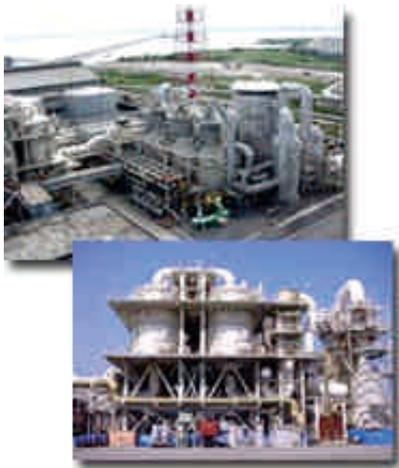
1. The SO<sub>2</sub> gas from smelter is cleaned from the dust in the washing tower, ventury scrubber, gas Coolers and mist precipitators.
